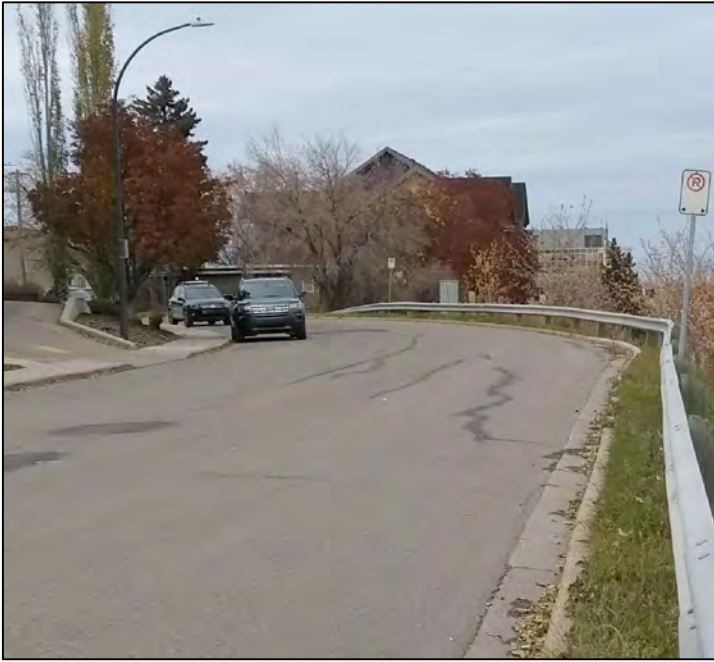
PHOTOGRAPH 7 (2018): SEALED CRACKS AND ROTATED GUARD RAIL ON SERVICE ROAD AT THE CREST OF SLOPE, FACING NORTH
