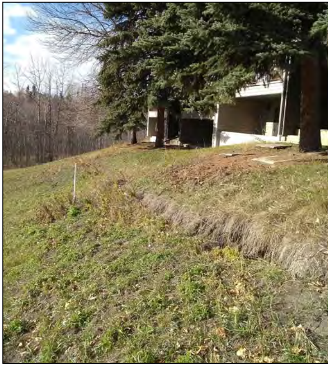
PHOTOGRAPH 16 (2018): TENSION CRACKS ALONG CREST OF 1982 LANDSLIDE SLOPE, FACING NORTHWEST
