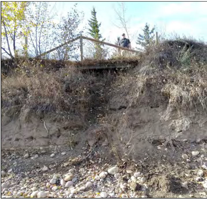
PHOTOGRAPH 84 (2018): WASHOUT AND UNDERMINING PEDESTRIAN TRAIL, FACING WEST
