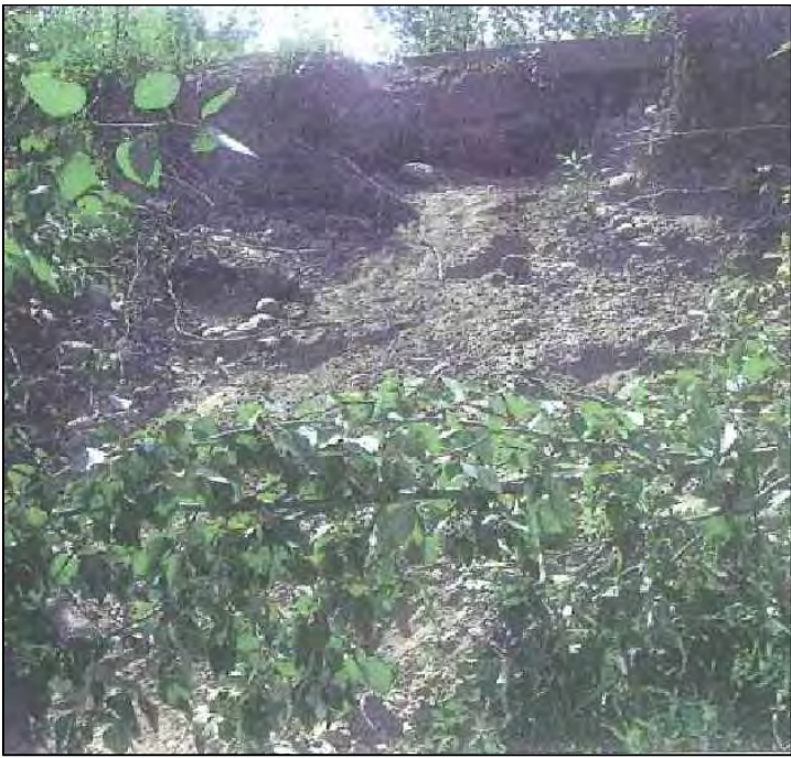
PHOTOGRAPH 84 (SHORTLY AFTER 2006 FLOODING): WASHOUT AND UNDERMINING PEDESTRIAN TRAIL AT NORTH END OF STUDY AREA 3, TAKEN FROM RIVER BACK TOE FACING WEST
