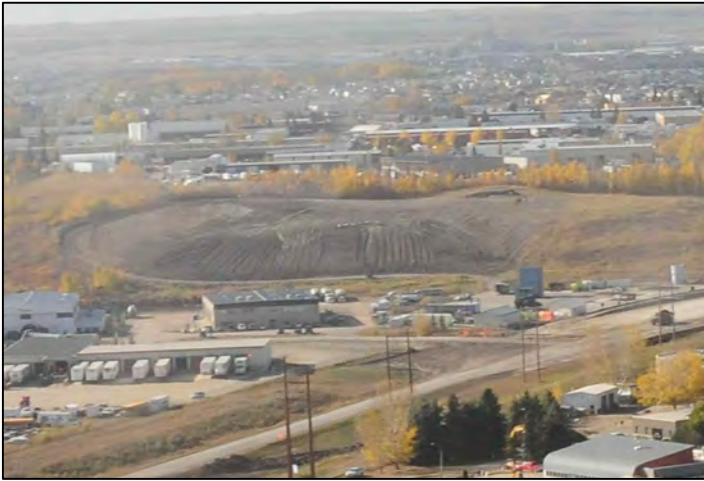
PHOTO 20 (2011): REMEDIATED SLOPE SHORTLY AFTER CONSTRUCTION, TAKEN FROM AERIAL LOCATION OVER RED DEER RIVER, FACING WEST
