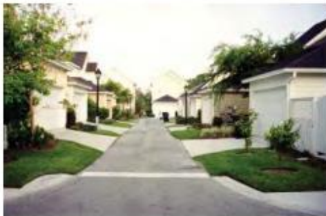
Lane Treatment - Design Elements: Garbage collection route with narrow pavement width, Asphalt paving.
