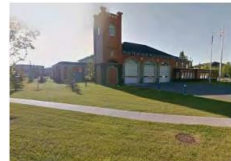
Mackenzie Towne Fire Station
