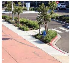
Coloured concrete in median paving area.
