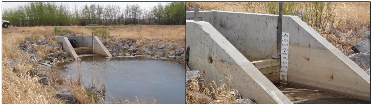
Photo 2: Hazlett Lake Gauge Station
