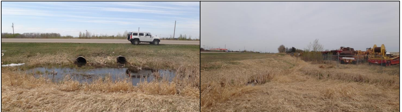
Photo 4: Highway 2A Culvert Crossings and Downstream Ditch
