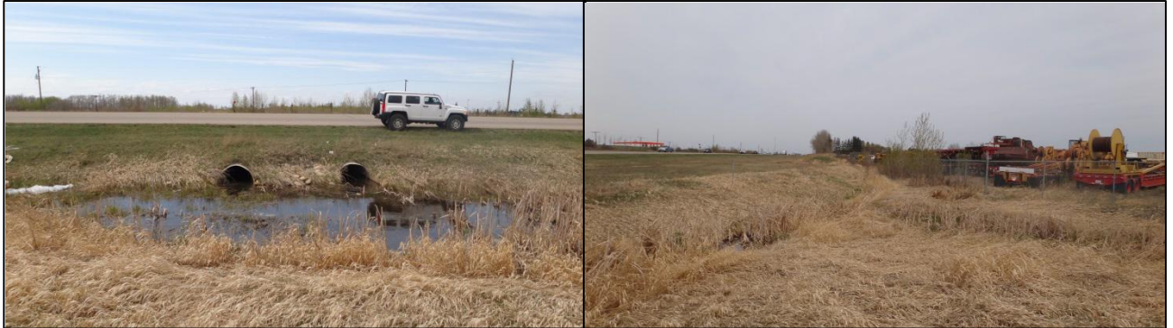
Photo 4: Highway 2A Culvert Crossings and Downstream Ditch
