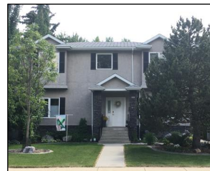
Redevelopment – second storey addition
