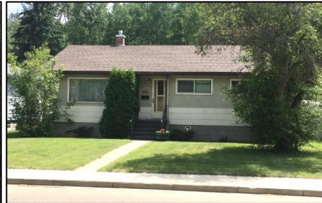
Typical Ranch style dwelling with Gable Roof Consistent Roof Design
