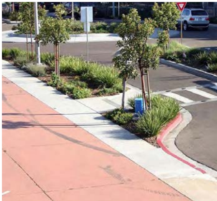
Coloured concrete in median paving area.
