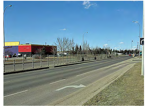
Existing fence along Taylor Drive median
