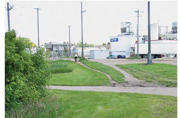
Existing south end termination of old CPR bridge (view from south of bridge)
