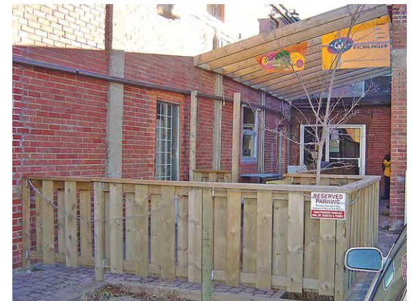
A flourishing group of businesses opening onto the back lane (North of Ross St.)
